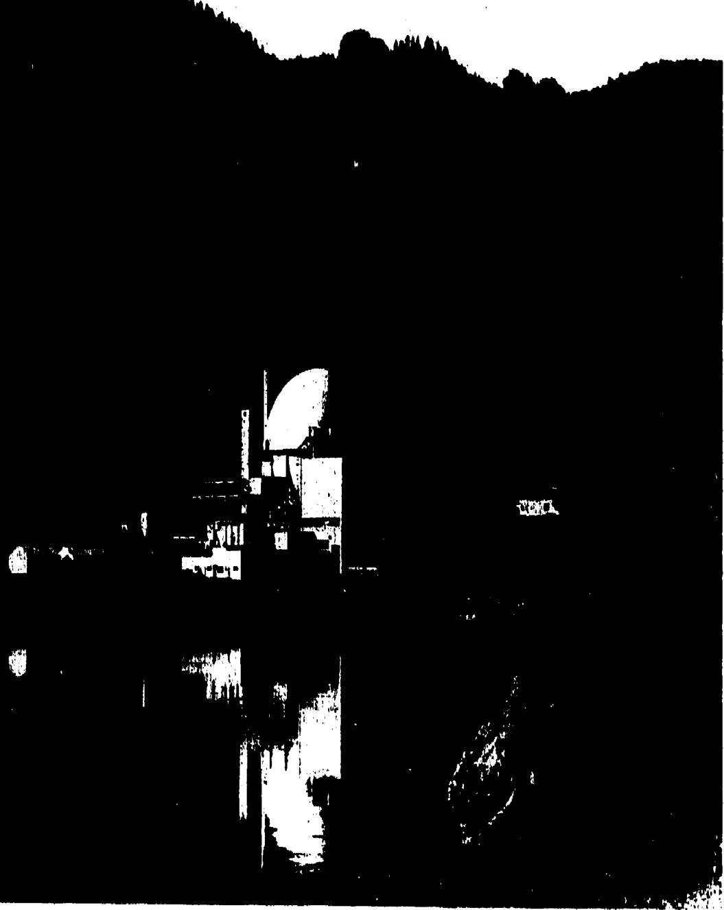
The Yankee Nuclear Power Station.
