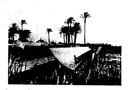
Figure 13 In 1913, the Shuman-Boys solar power plant in Meadi, Egypt, was successfully powered by solar steam along the banks of the Nile River.
