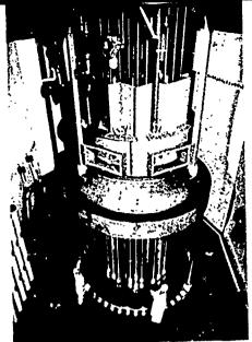
Figure 10 Reactor vessel head being installed at a nuclear power plant.
