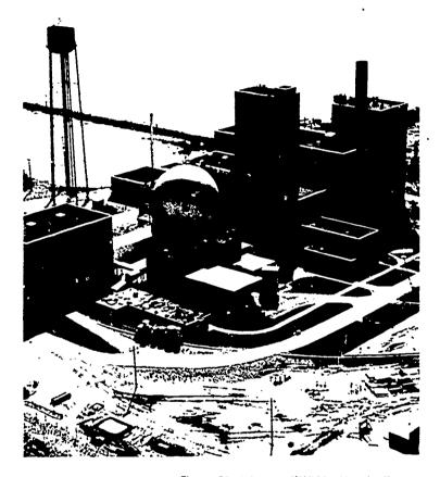
Figure 21 ENRICO FERMI Atomic Power Plant. Located at Lagoona Beach on Lake Eric, near Monroe, Michigan, about 35 miles southwest of Detroit. Breeder reactor, cooled with liquid sodium, 60,900-net-electrical-kilowalt capacity, designed by Atomic Power Development Associates, Inc. Started power operation in 1905. Jointly owned and operated by Detroit Edison Company and Power Reactor Development Company. Envico Fermi was the world's first large breeder nuclear power plant.
