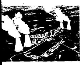
Figure 34 England's CAL-DER HALL Suclear Power Station. The tall structures are cooling towers, which are employed in locations where a large body of water is not accessible. These towers cool the condenser cooling water so that it can be used again, and they emit steam, not smoke. Four reactors subply steam to two turbines. Total capacity of the station is 198,000 electrical kilowalls.
