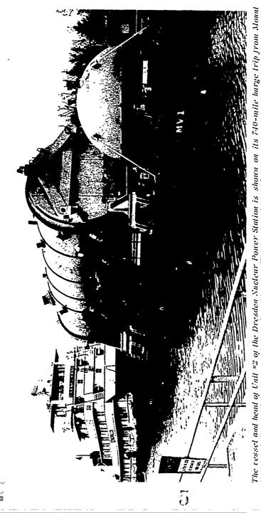
The vessel and head of Unit #2 of the Dresden Nuclear Power Station is shown on its 740-mile barge trip from Mown Vernon, Indiana, where it was fabricated, to Morris, Illinois. It weighs 800 tons and is approximately 72 feet tong and 22 feet in diameter. (See Figure 18 on page 28.)
