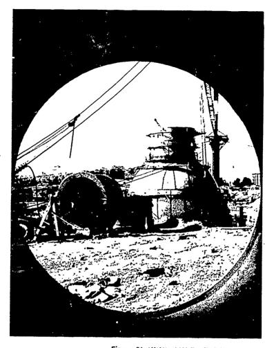
Figure 31 NINE MILE POINT Nuclear Station, under construction. It takes seteral years time, a lot of material, and many hours of tabor to erect a targe power plant. In taking this pictare, the photographer stood inside a targe pipe that carries cooling water from Lake Ontario onto the steam condenser. The hage, light-bulb-shaped steel shell in the foreground houses the reactor. A view of the finished plant is shown in Figure 32.
