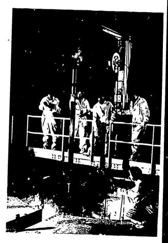
Figure 12 Lowering a fuel assembly into a reactor core.
