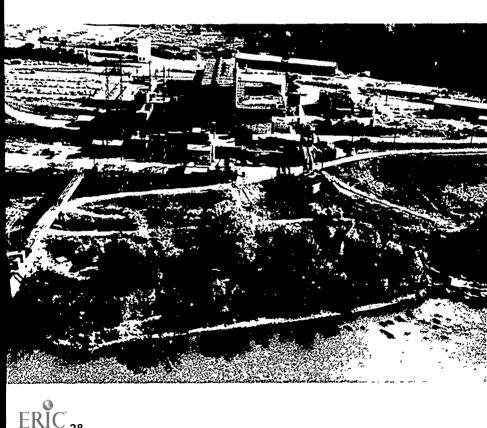
Figure 18 DRESDEN Nuclear Power Station, Unit #1, Located at Morris, Illinois, about 50 miles southwest of Chicago, Boiling-uater reactor, 200,000-net-electrical-kilouatt capacity, designed by General Electric Company, Started commercial operation in 1969, Owned and operated by Commonwealth Edison Company, Dresden Unit #1 was the second large nuclear power plant to be built in the U.S. Dresden Unit \$2 and Unit #3 adjoin Unit #1. (See frontispiece.)
