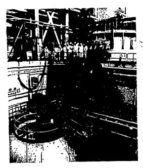
Figure 39 The reactor (nt in the NOVOVORONEZH Nuclear Power Station located on the Don River in the Soviet Union. The dome at the bottom is a cover for the reactor vessel. This plant produces 196,000 kilowatts; a second, larger plant is at the same sile.
