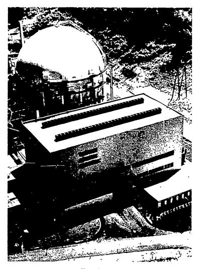
Figure 19 YANKEE Nuclear Power Station. Located at Rowe, Massachusetts, about 45 mites east of Albany, New York. Pressurized-water reactor, 175,000-net-electrical-kilowatt capacity, designed by Westinghouse Electric Corporation. Started commercial operation in 1961. Ouned and operated by Yankee Atomic Electric Company. Yankee was the third large nuclear power plant to be built in the U, S.
