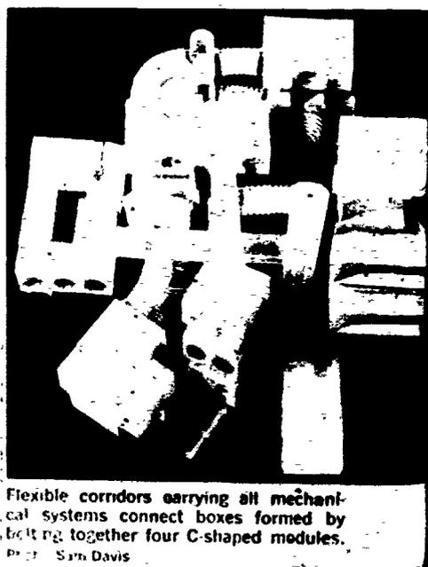
Flexible corridors carrying all mechanical systems connect boxes formed by bolting together four C-shaped modules.
