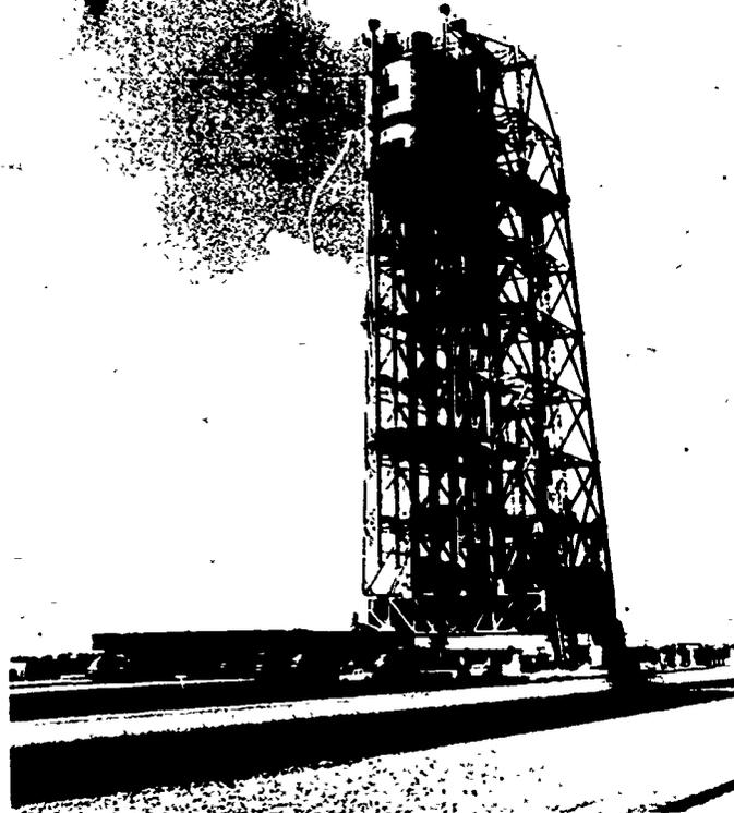
Figure 7. Mobile service structure.
