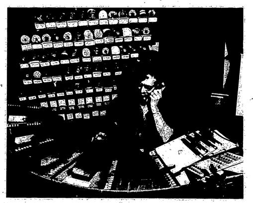
Fig. 2. Telephône Dial Access Library: Operator receiving call to Wisconsin Dial Access Library places appropriate cartridge in the playback unit, presses a button to connect the unit with the telephone line, and is then ready for the next call while the tape plays to its conclusion. Five callers may be served simultaneously from the library
